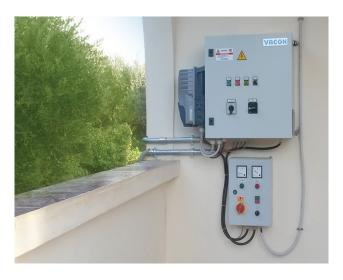
VACON 100 X installed outdoors to control solar-powered water pump system. VACON 100 X has dedicated functionality to drive the solar-powered pump with an optimized efficiency.
